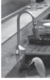
ECR-D0810-107 modified with B-0107-C Spray (0.65 GPM)
